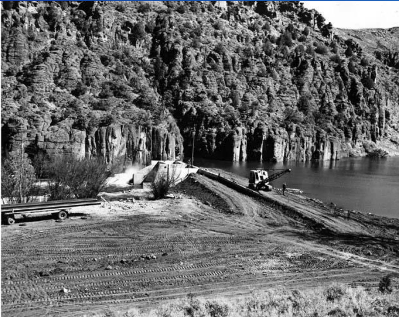
P549-100-973 A privately-constructed low dam was put across the Teton River in 1960-61 by Mr. Lindermann. The purpose of the dam is to develop hydraulic pumping power to lift irrigation water to Mr. Lindermann's farmland lying along the south canyon rim. This dam is below the north fork of the Teton River. Teton Basin Project, ID. FACI/Other Structures. BR photo by D.L. Crandall. Spring 1961.
