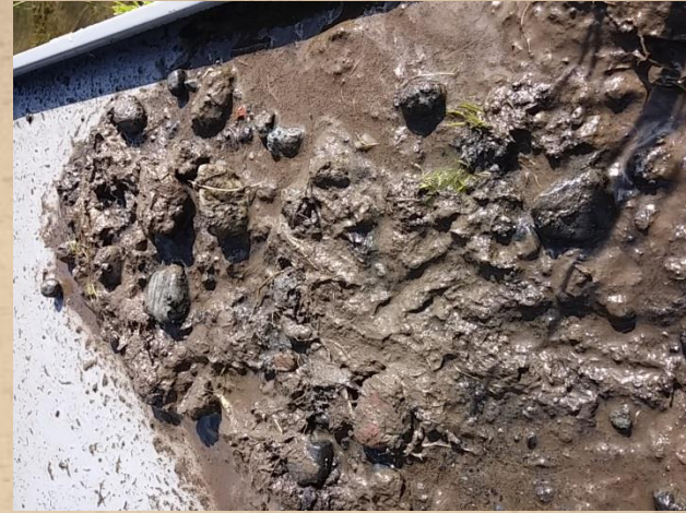
Downstream of culvert
