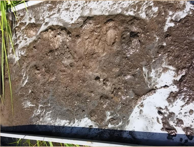
Upstream of culvert
