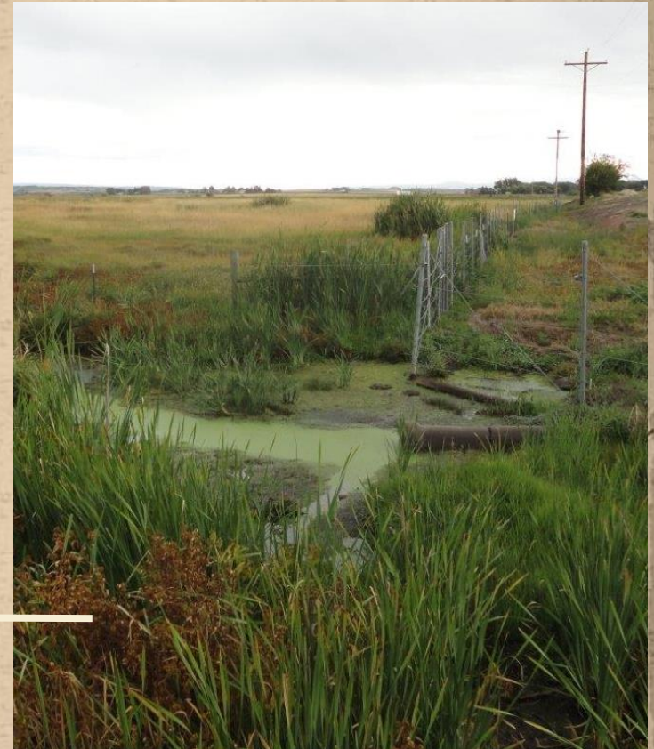
EPA photo, Sept. 2013 Plant not discharging
