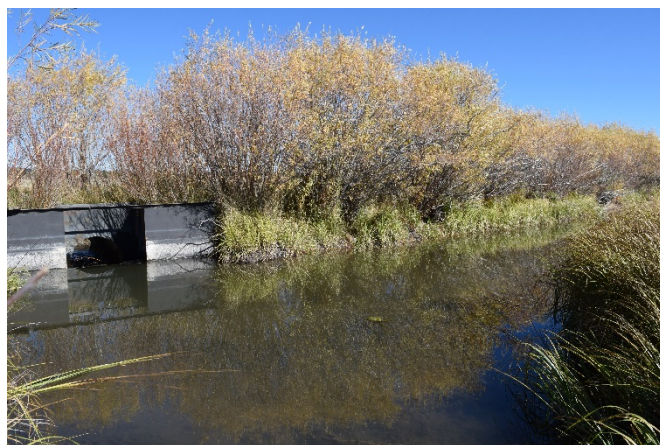
Figure 4. Second return flow point.
